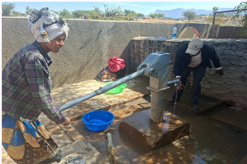
Figure 5: shallow well, Adigobye Carnevali School, phase 1 drilled
