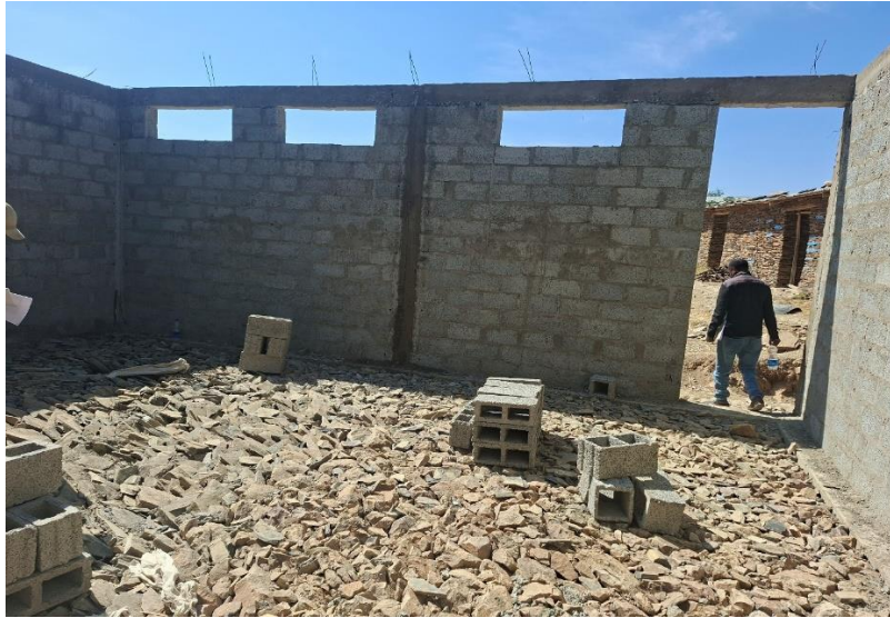
Figure 1: Hard core, Adigobye school, view from interior to front gate
