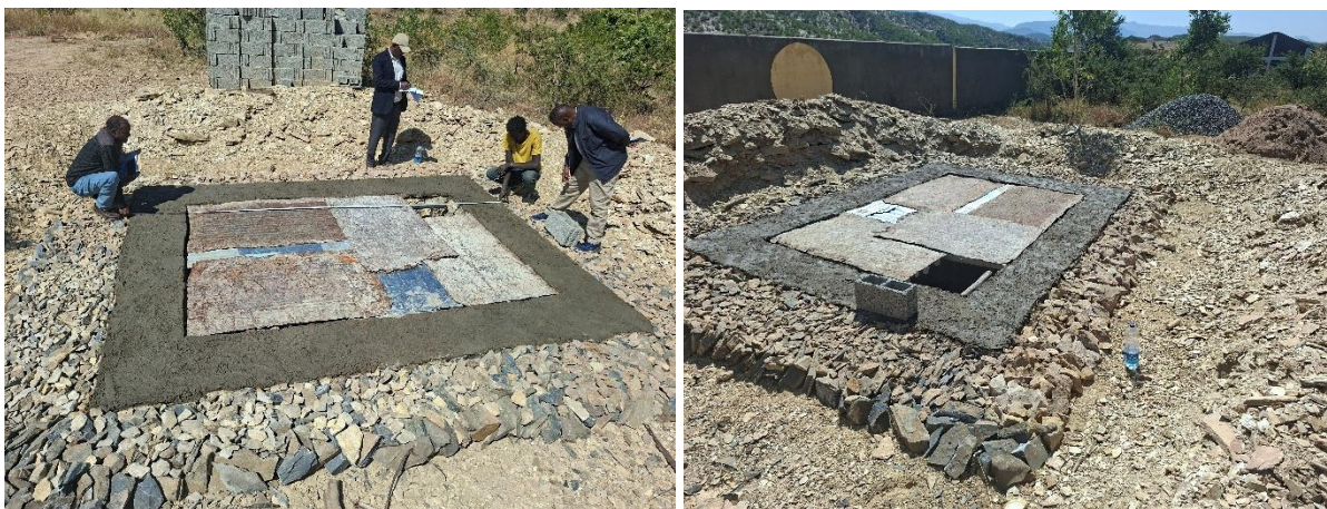
Figure 4: New toilet excavation, underground mason and formwork for slab
