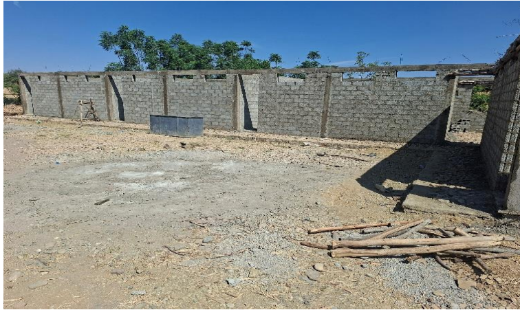
Figure 3: Adigobye phase 2, classrooms front view
